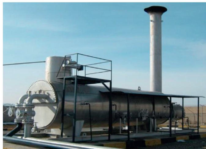
Fig. 1. A typical indirect water bath heater: (a) schematic diagram and (b) real photograph [28].
